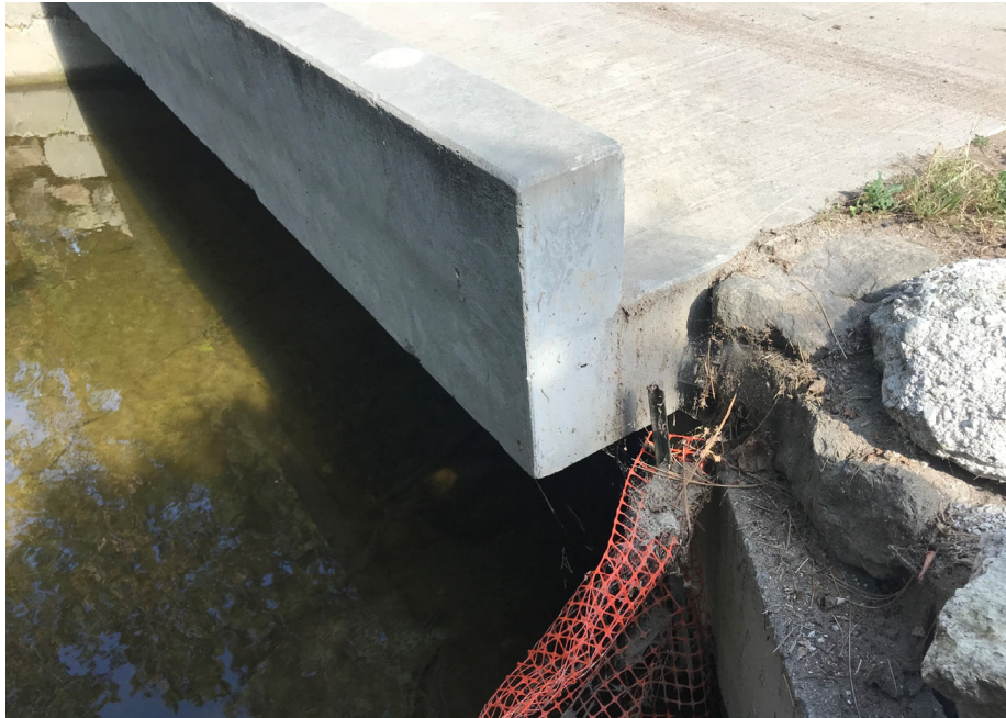
South exterior stringer not bearing on east abutment
