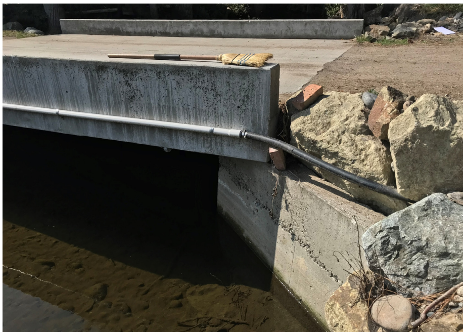
Northwest wingwall – cold joint and honeycombing
