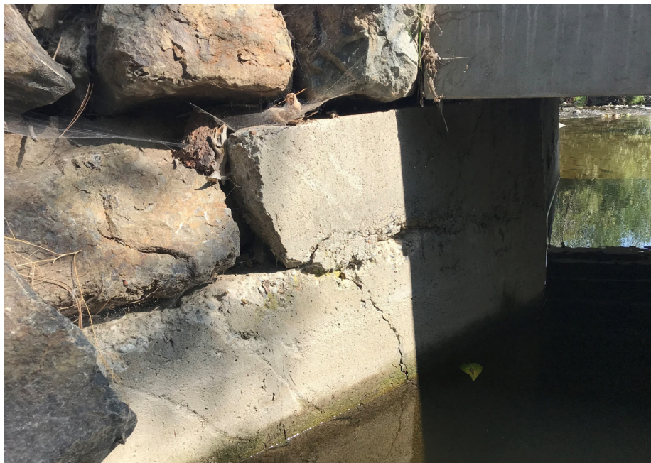
Southwest wingwall – note wide vertical crack and horizontal cold joint
