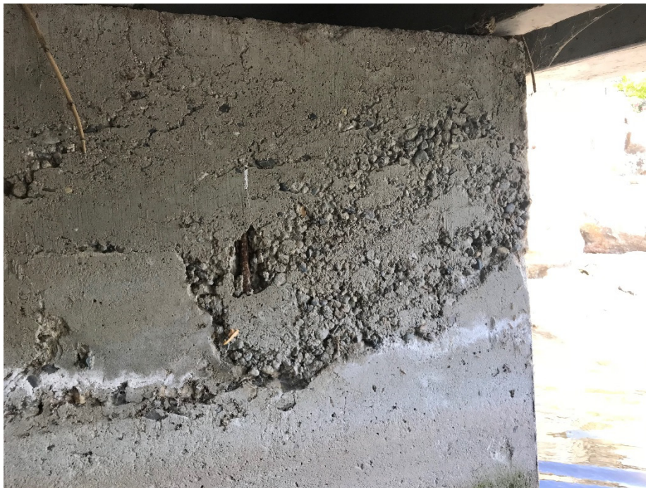
West abutment – honeycombing, exposed reinforcing
