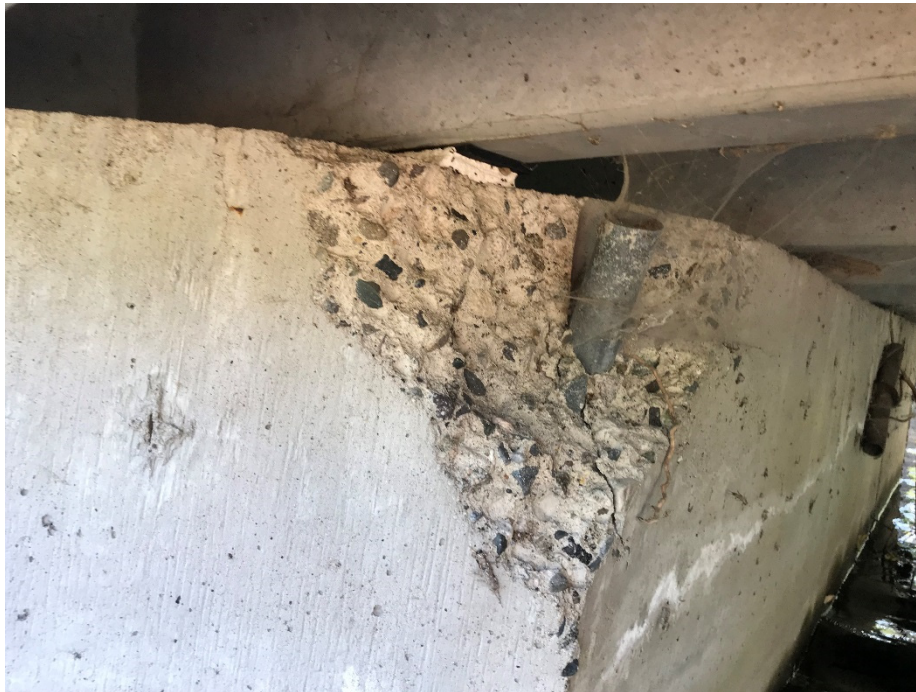
East abutment – spall with galvanized pipe
