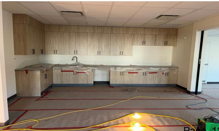
Kitchen cabinets - altered to allow space for coffee machines
