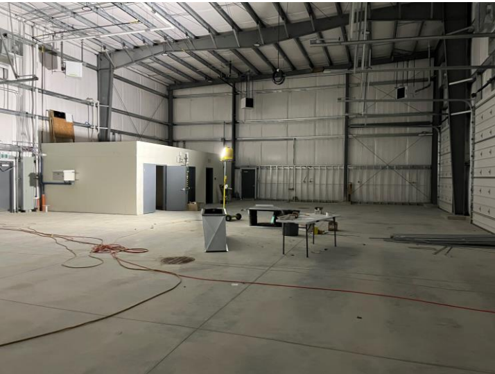
Interior main area
