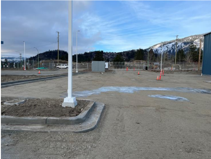
Grading complete from main entrance and between buildings, sub-base installed
