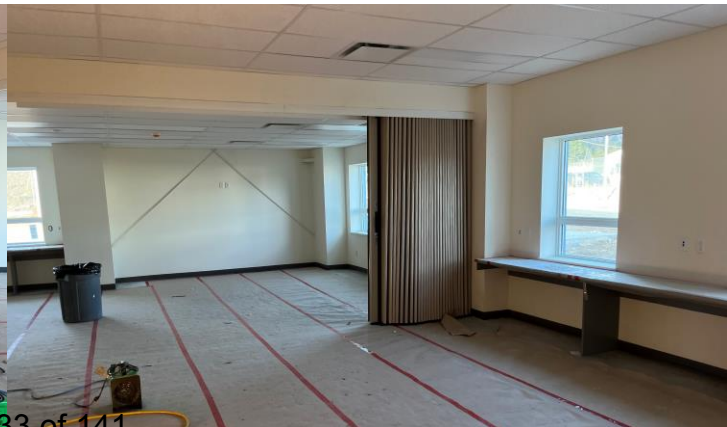
Lunch room/meeting room with dividing wall installed
