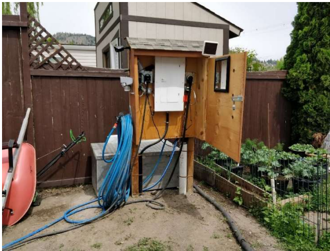
Figure 1 – Service Connections and Electrical Panel
