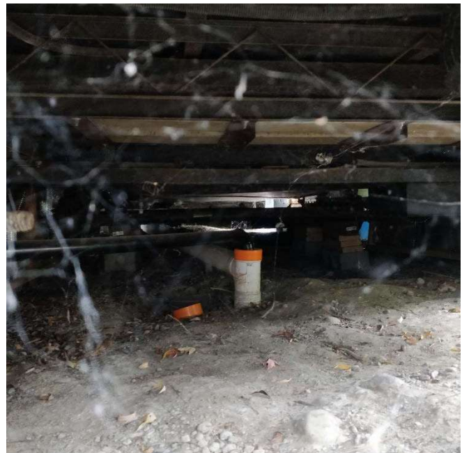
Figure 4 – View of Sanitary Connection under RV
