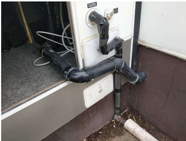
Figure 3 – Water Connection into RV and Sanitary
