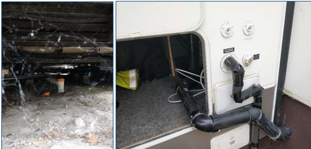
Figure 2 - Sanitary Service Connection
