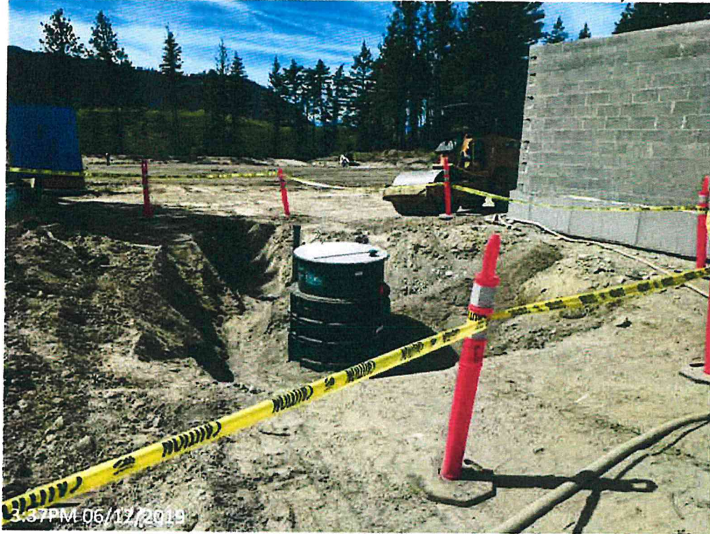
Figure 1 – Sanitary Sewer Lift Station Installed (East of washroom)
