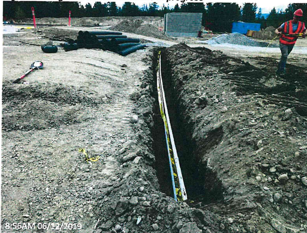
Figure 3 – Irrigation line installations in progress
