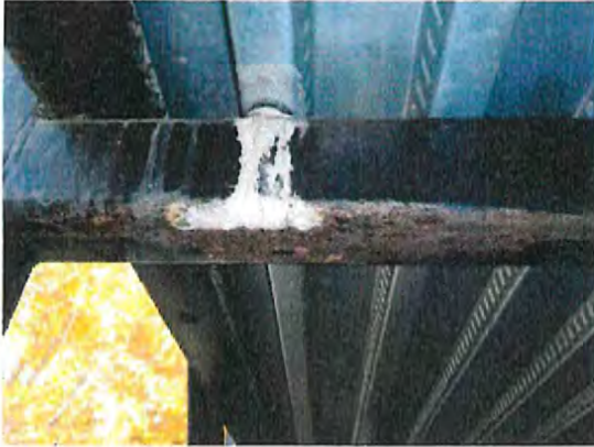
Coating (Struct): Note localized light corrosion with no section loss
