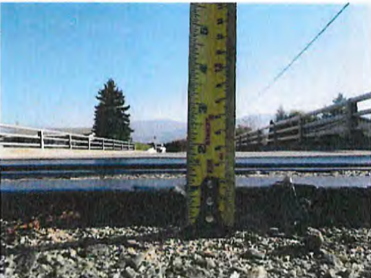
Deck Joints: 38mm gap and 25mm grade differential at West deck joint. 28mm gap at East deck joint. East angle plates minor debonding across 75% for deck width.
