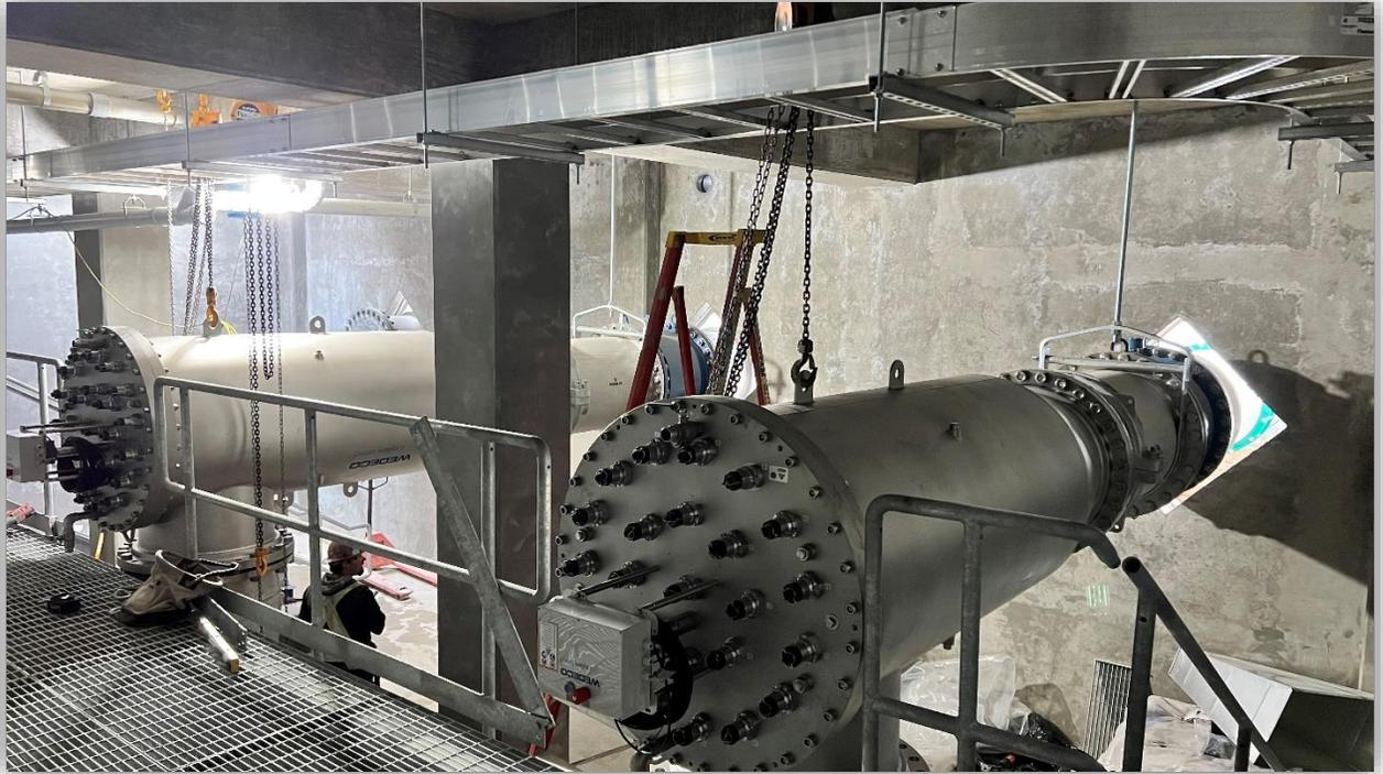
**Figure 2: Ultraviolet Disinfection**
