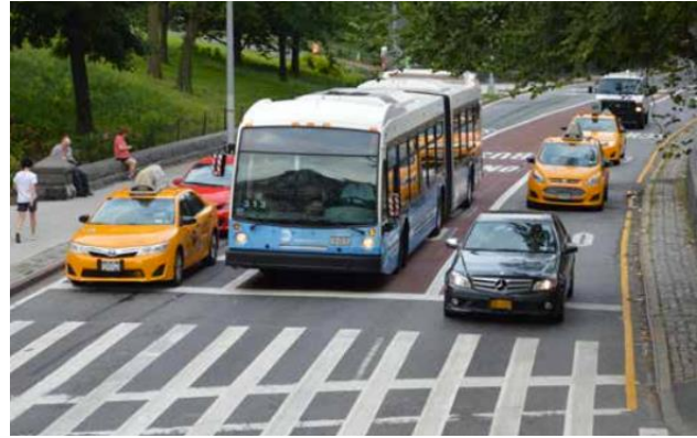
Figure 6: Transit queue jump lane at an intersection
