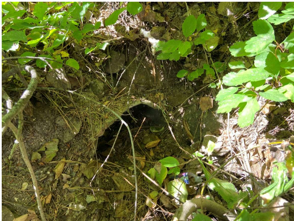
Photo 6: East culvert under Gill Road (~300mm CSP)
