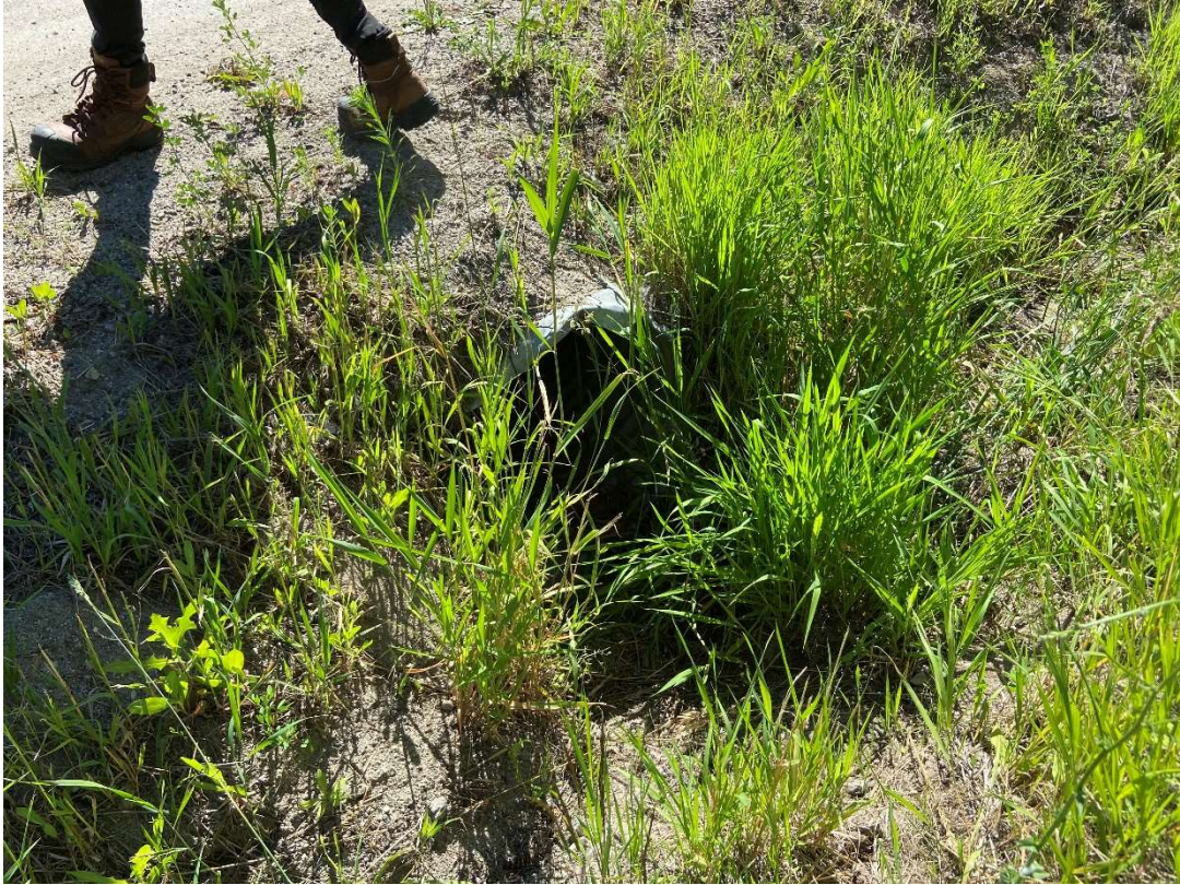
Photo 9: Culvert under Turnbull Road at Glenrosa Road
