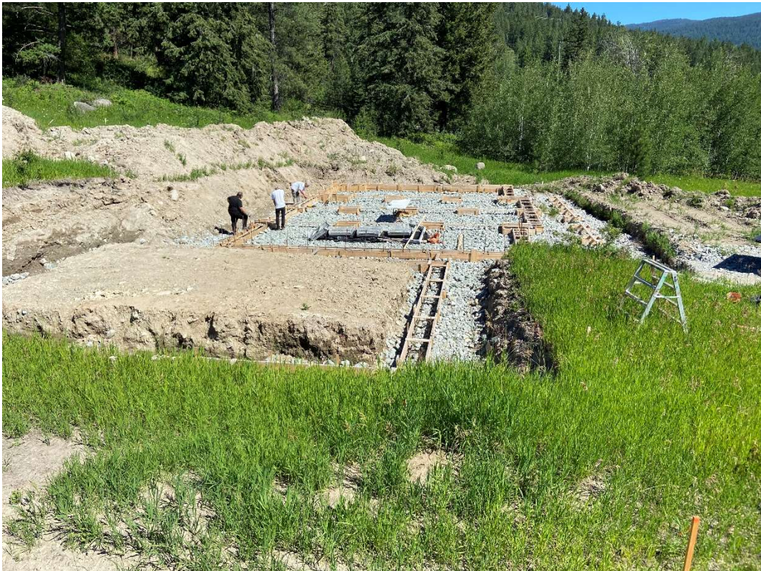
Photo 10: Footing forms on top of crushed stone
