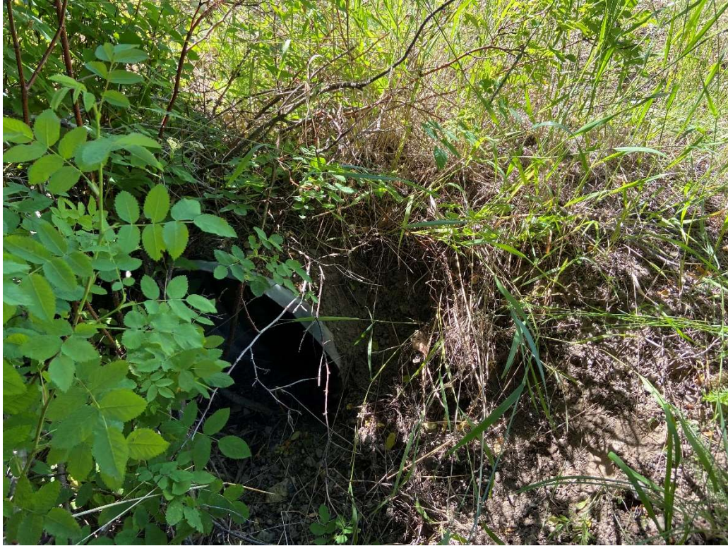
Photo 7: West culvert under Gill Road at McKeller Road (~600mm CSP)
