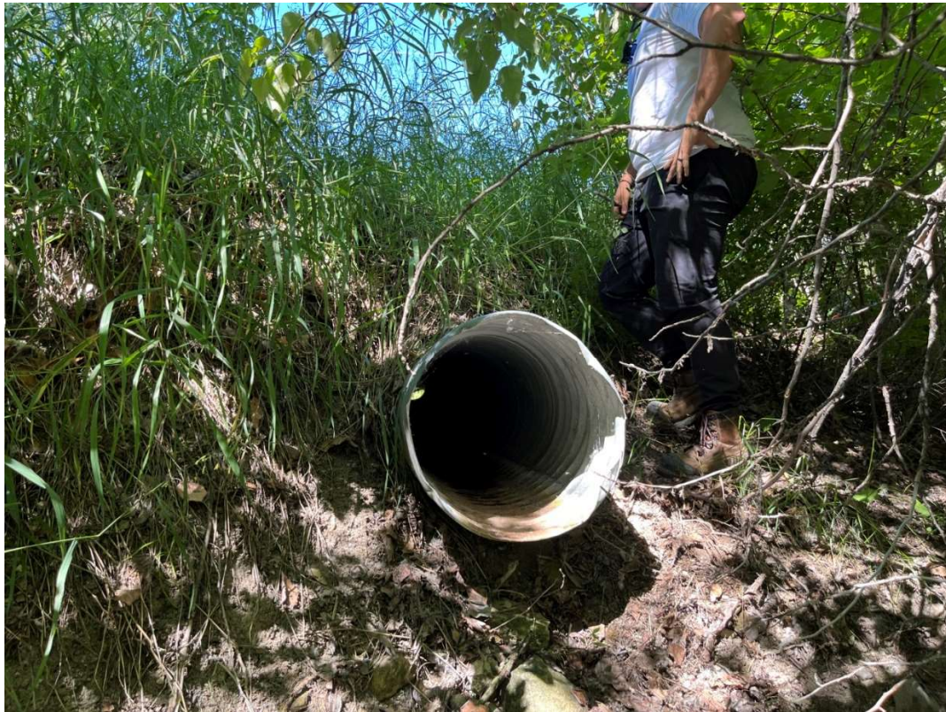
Photo 8: Culvert under McKeller Road (~600mm CSP)
