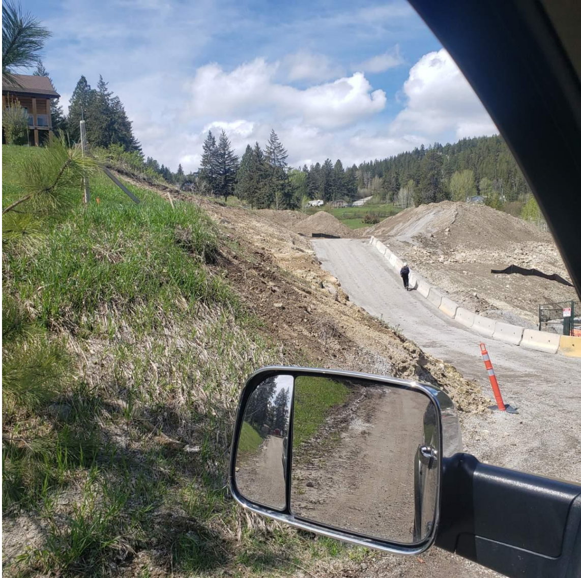
Figure 2: Looking West across the property
