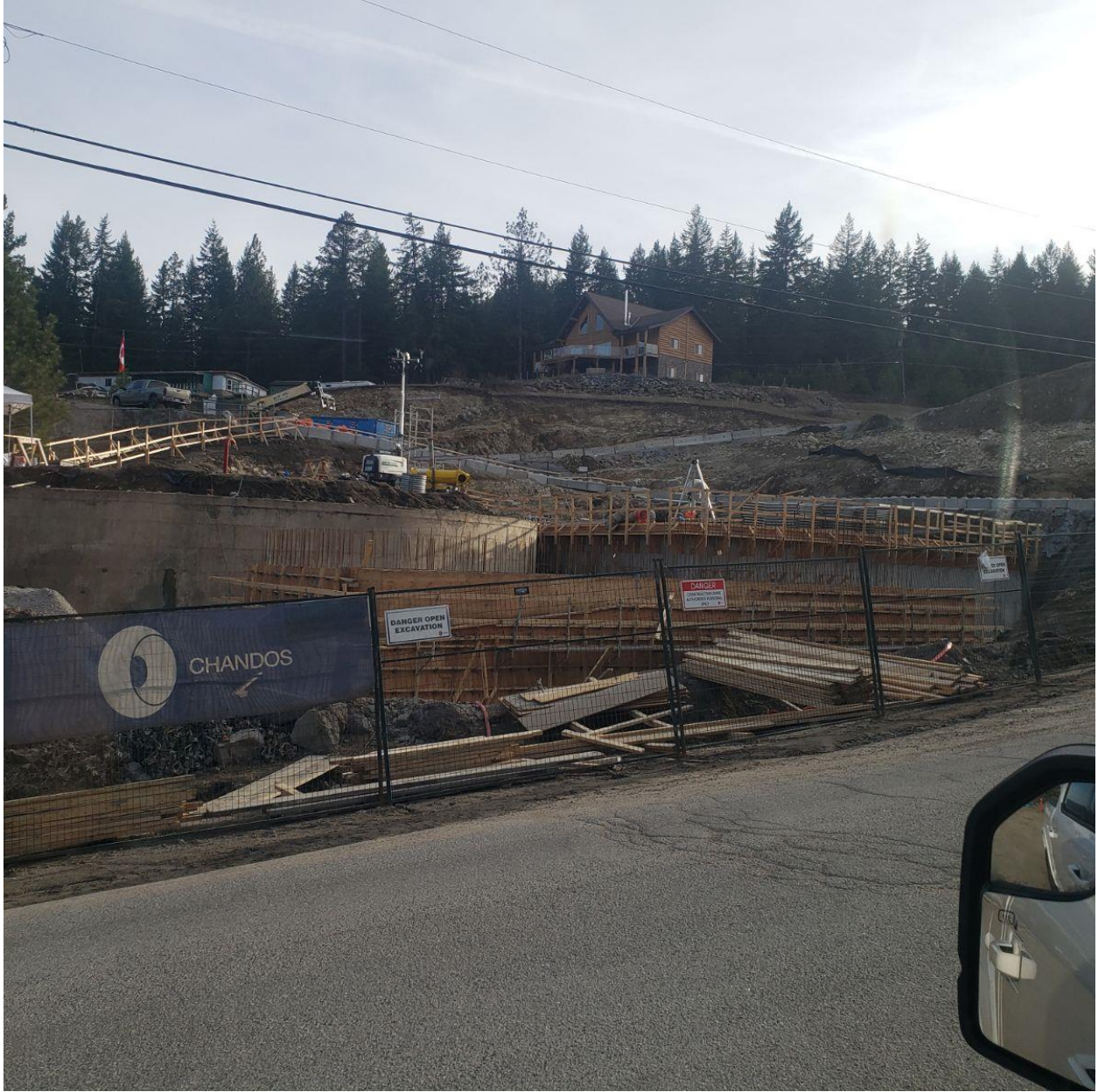
Figure 5: Current View from Glenrosa Road
