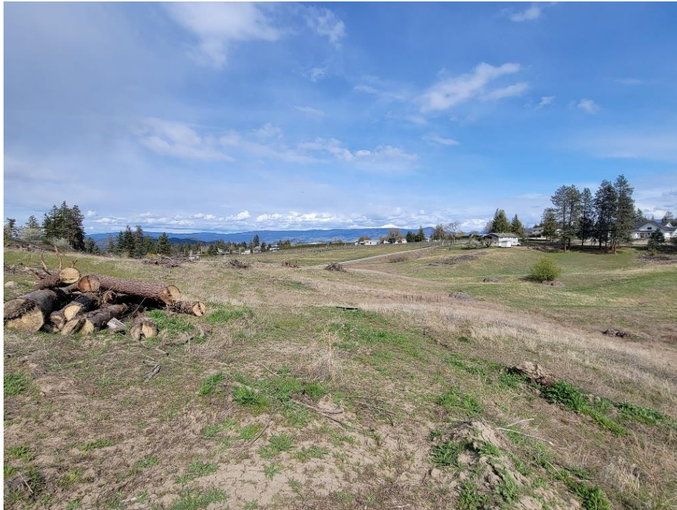
Photo 3. View facing east including log piles from recent clearing, at the northern extent of fill placement area.
