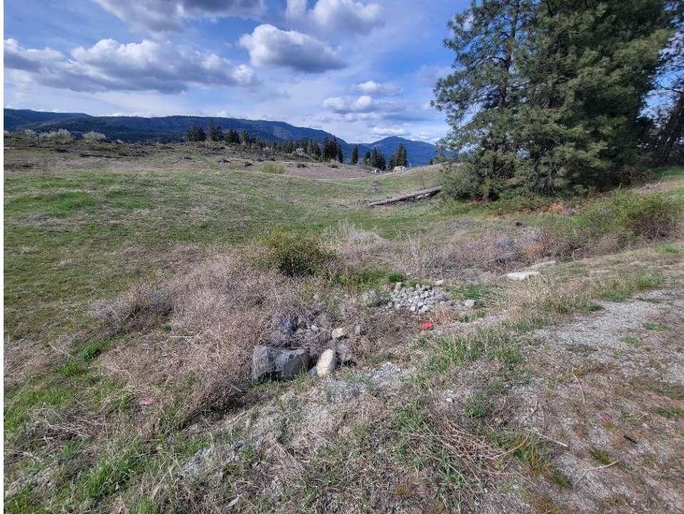
Photo 9. View facing northeast from Hayman Road of drainage swale constructed by the City of West Kelowna without landowner permission, proposed for redesign.
