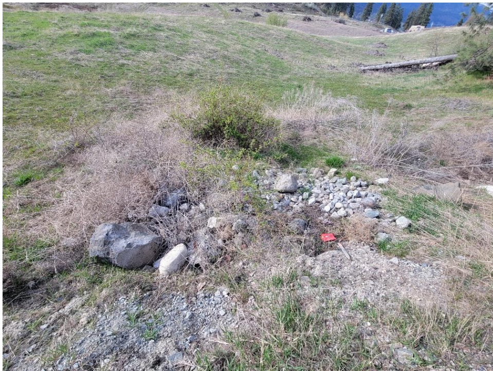
Photo 10. View of drainage swale proposed for redesign.
