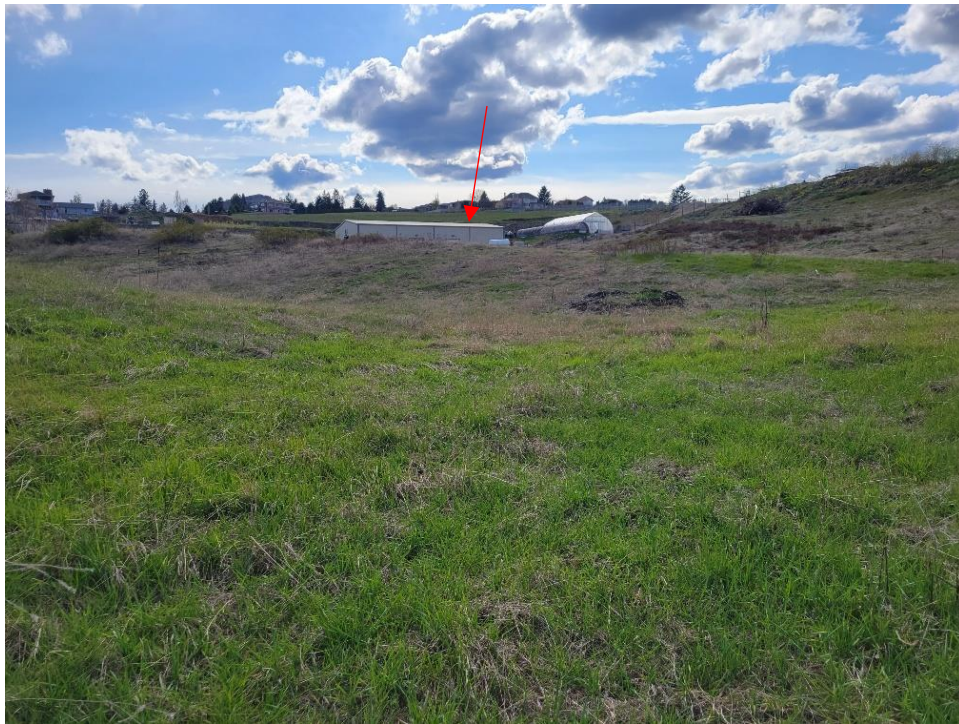
Photo 6. View facing west of Xen nursery (red arrow) and fill placement area.
