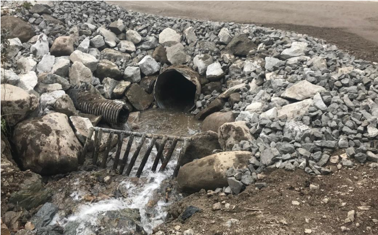
Photo 13: Project 13/26 – Rock Ridge Park – cleaned out culvert at Scott Crescent
