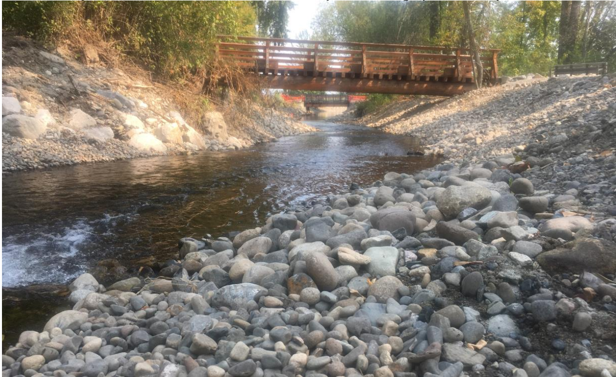
Photo 10: Project 19 – Lower Powers Creek – Rotary Bridge Post Recovery
