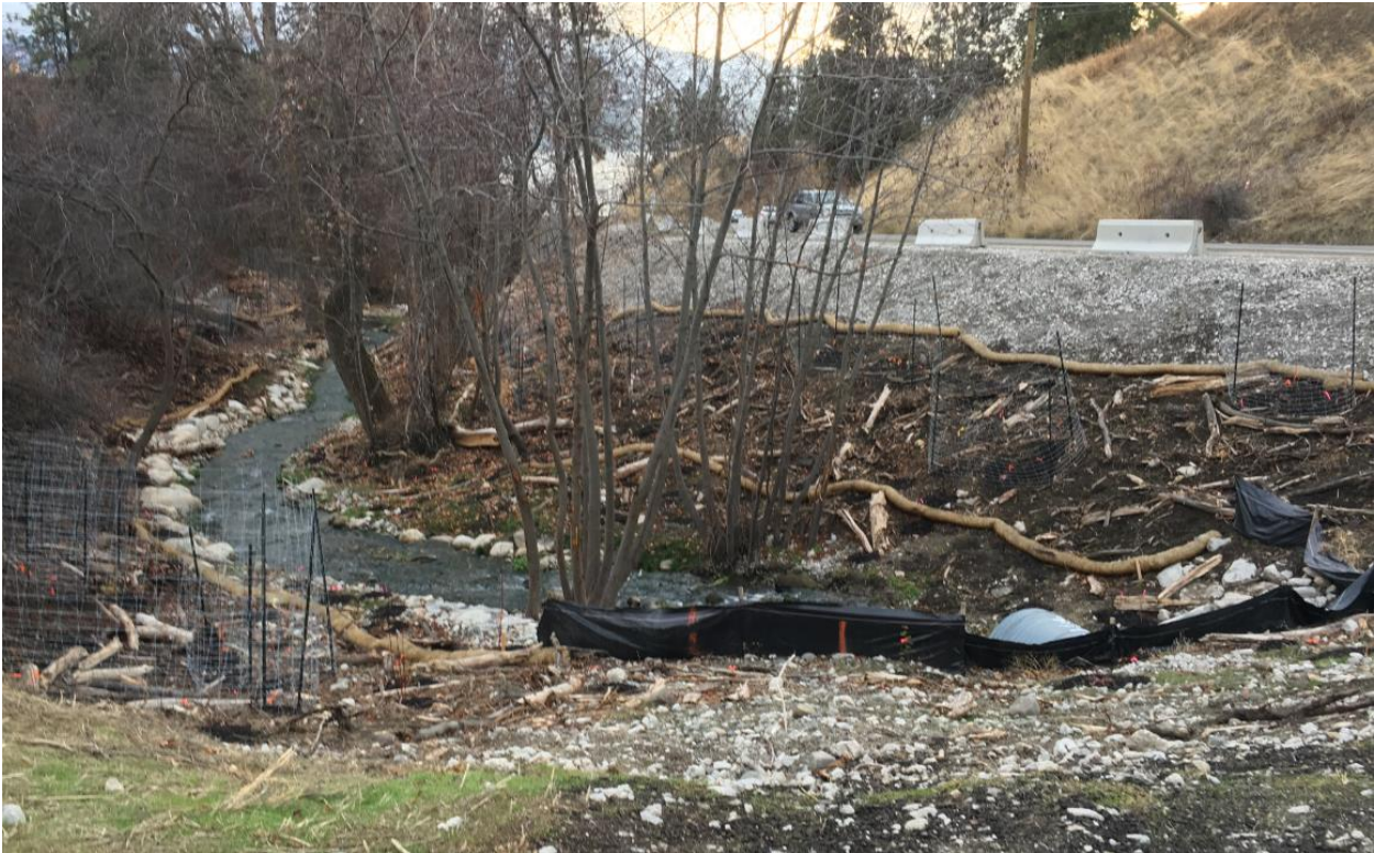
Photo 15: Project 34 – Smith Creek at Gellatly Road – bank stabilization
