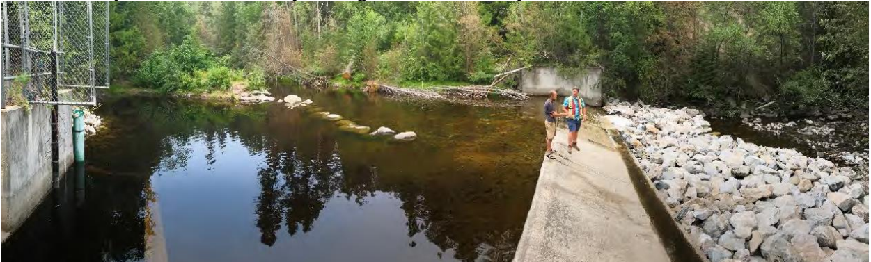
Photo 4: Project 14 - Rose Valley Headgate Post Recovery – south side of creek
