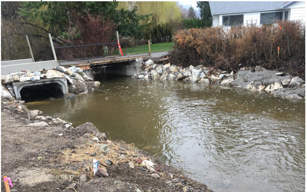
Photo 6: Project 18 - Lower McDougall Creek
