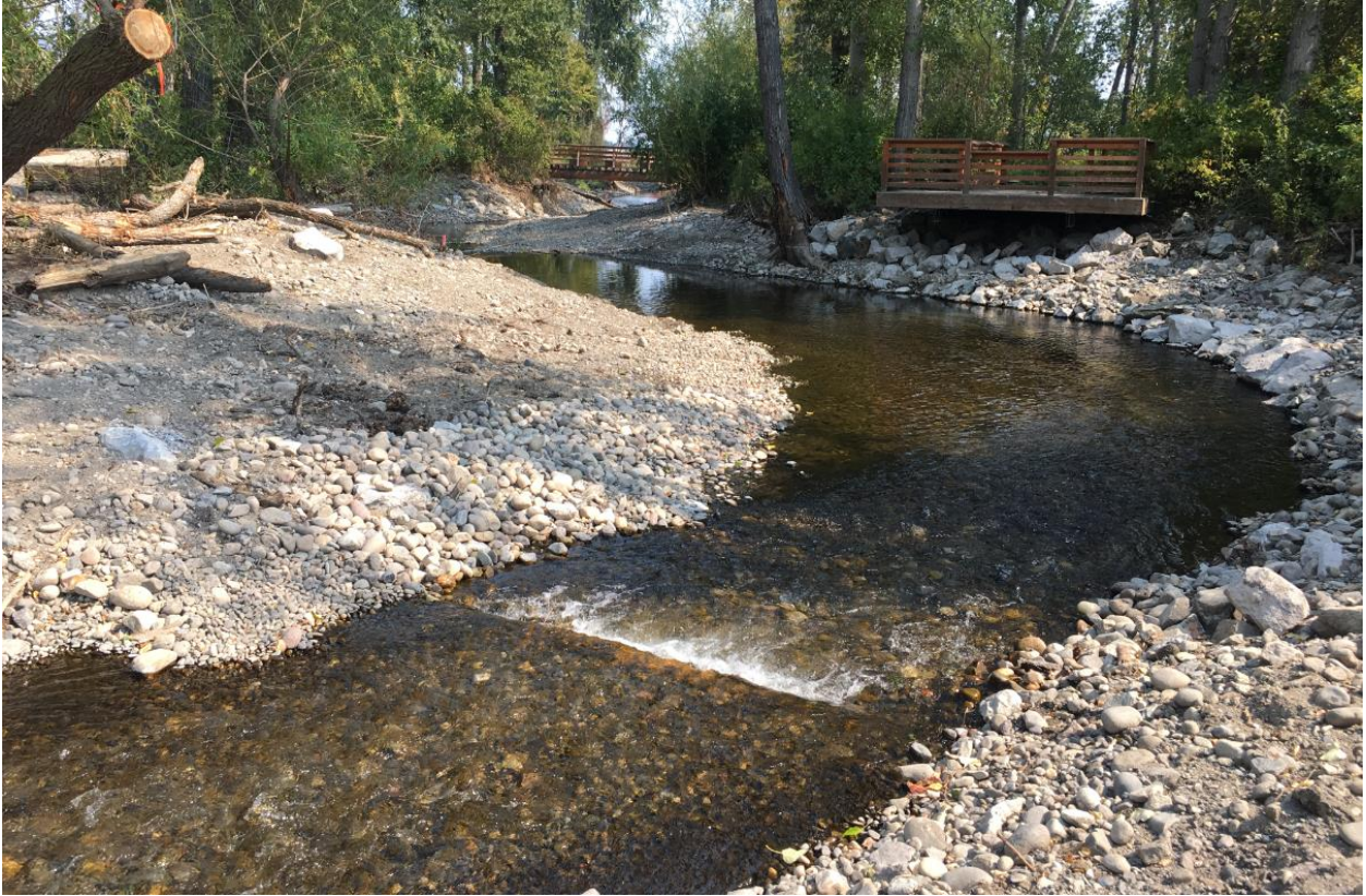
Photo 12 – Project 19 – Lower Powers Creek – creek channel re-established w/ fish habitat structures
