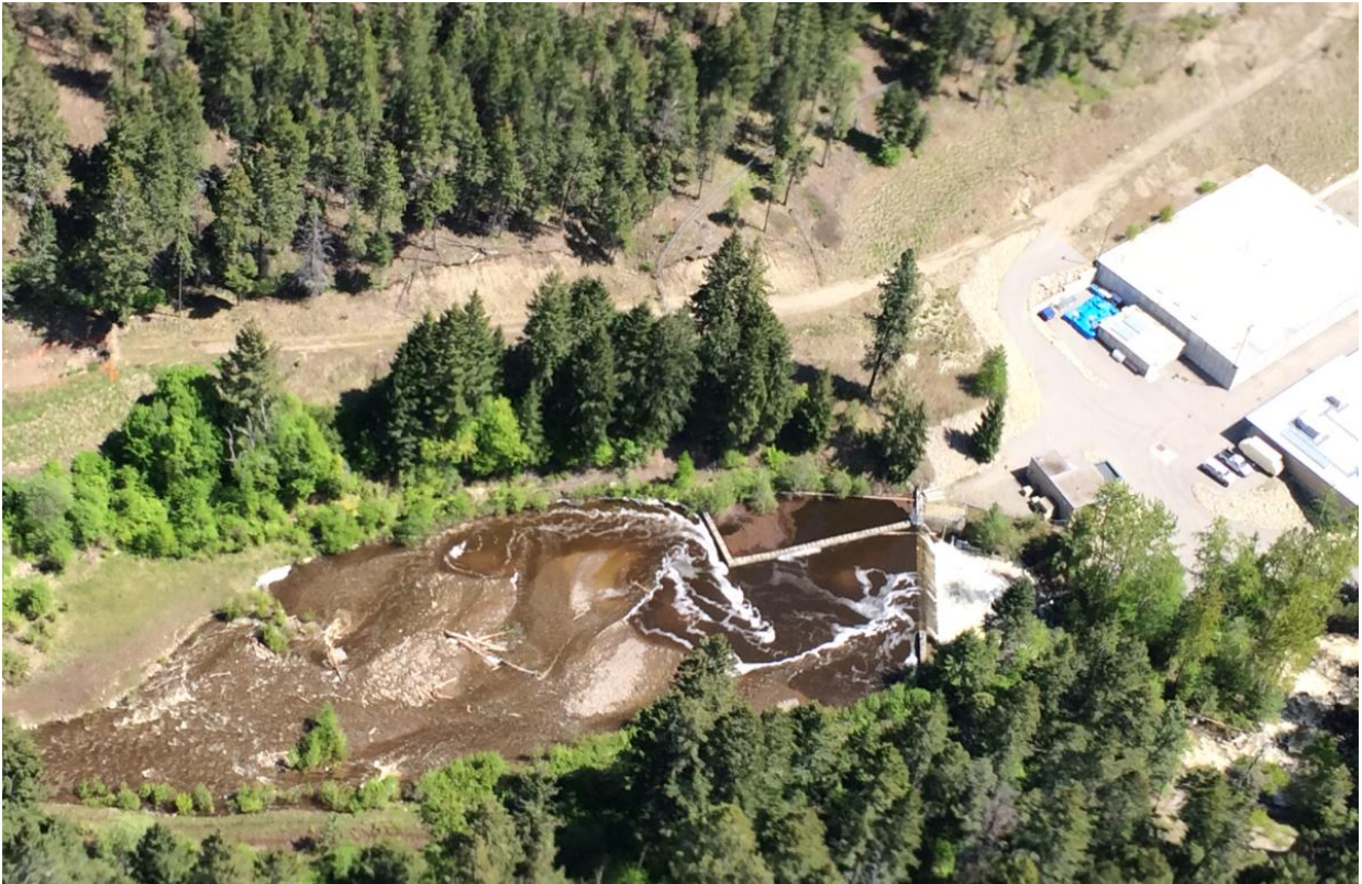
Photo 7: Project 19 - PCWTP - Pre-Recovery
