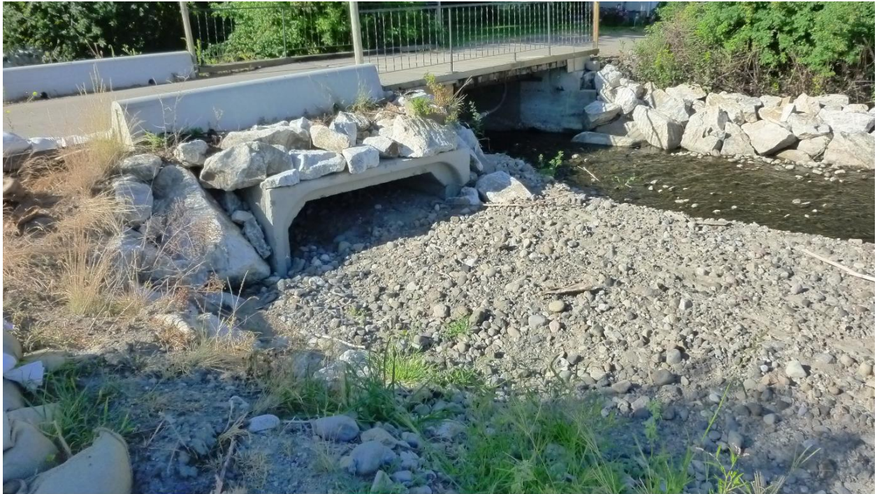
Photo 5: Project 18 - Lower McDougall Creek
