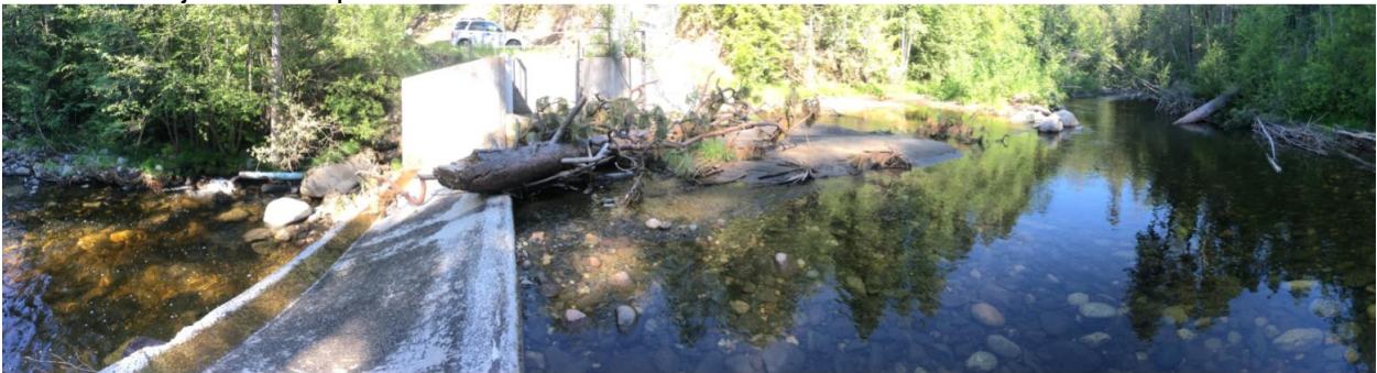
Photo 3: Project 14 - Rose Valley Headgate Pre-Recovery – north side of creek
