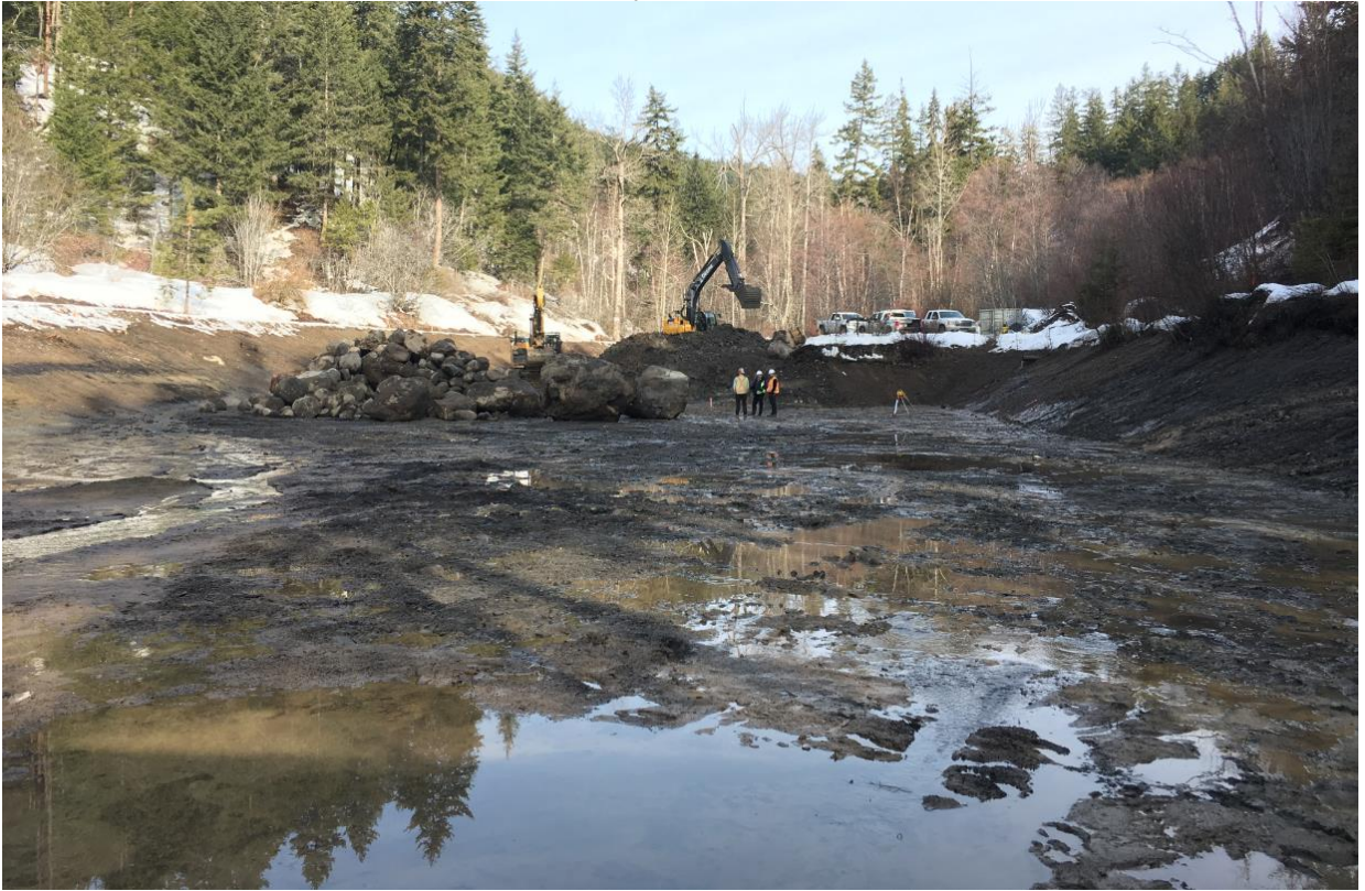
Photo 8: Project 19 - PCWTP - During Recovery
