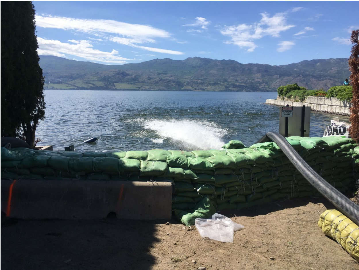
Example of pumping ground water out of the Green Bay neighbourhood.
