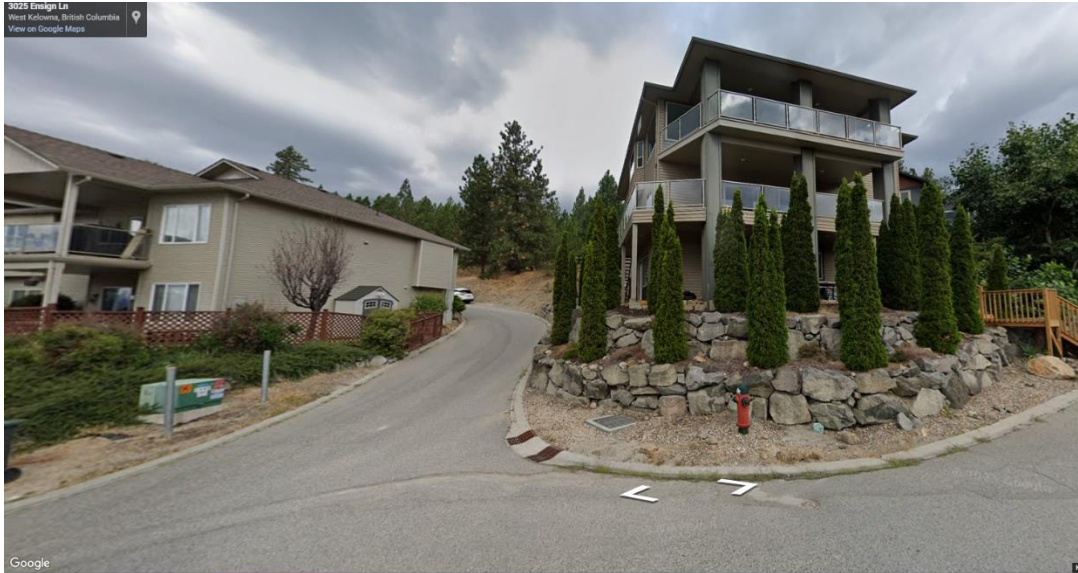
Figure 6b: Ensign Quay Lane access to units 21-38 (18 units) – ~5.6 m width is constrained by existing retaining wall and single family residence.
