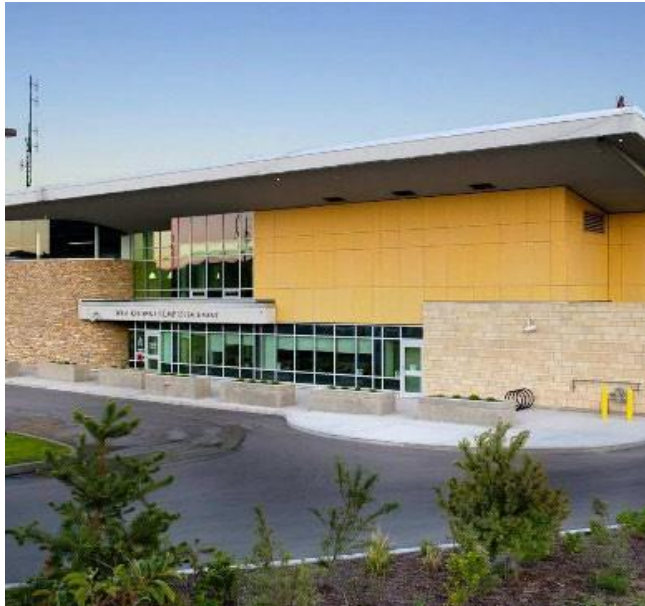
FIGURE 1 - RCMP LEED BUILDING
