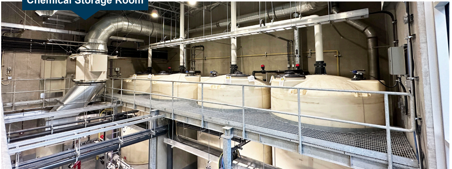
Chemical Storage Room
