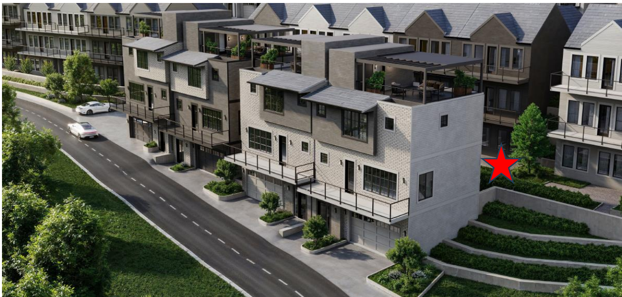
Figure 5: Units 55-58 fronting Ensign Quay Lane / along with pedestrian mews noted with a red star.
