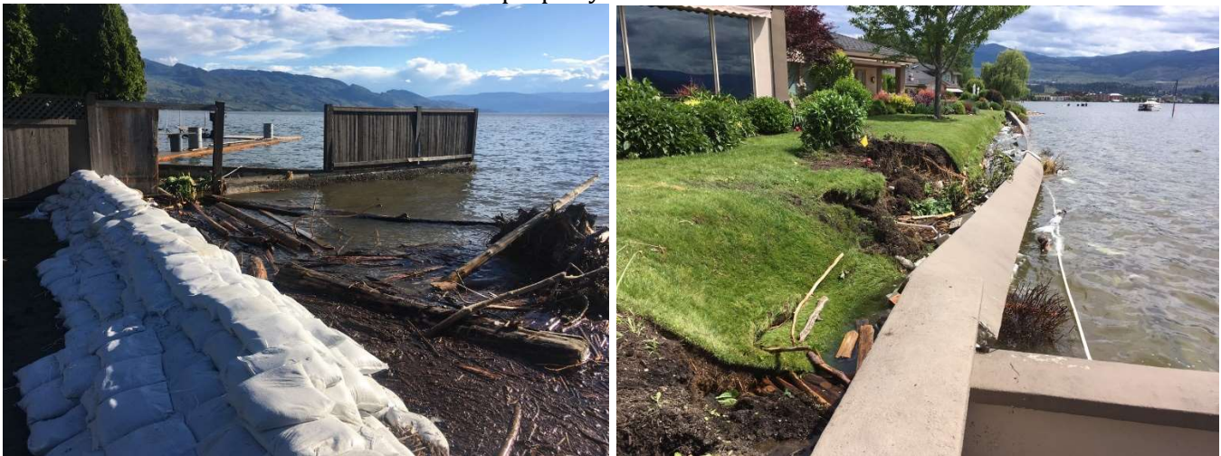
Figure 7 – Okanagan Lake 2017 Flood Damage Examples (Debris Impact and Wall Failure)
