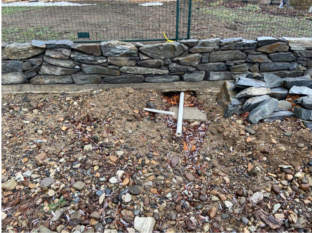
Photo 15: PVC pipe from lawn drain under retaining wall
