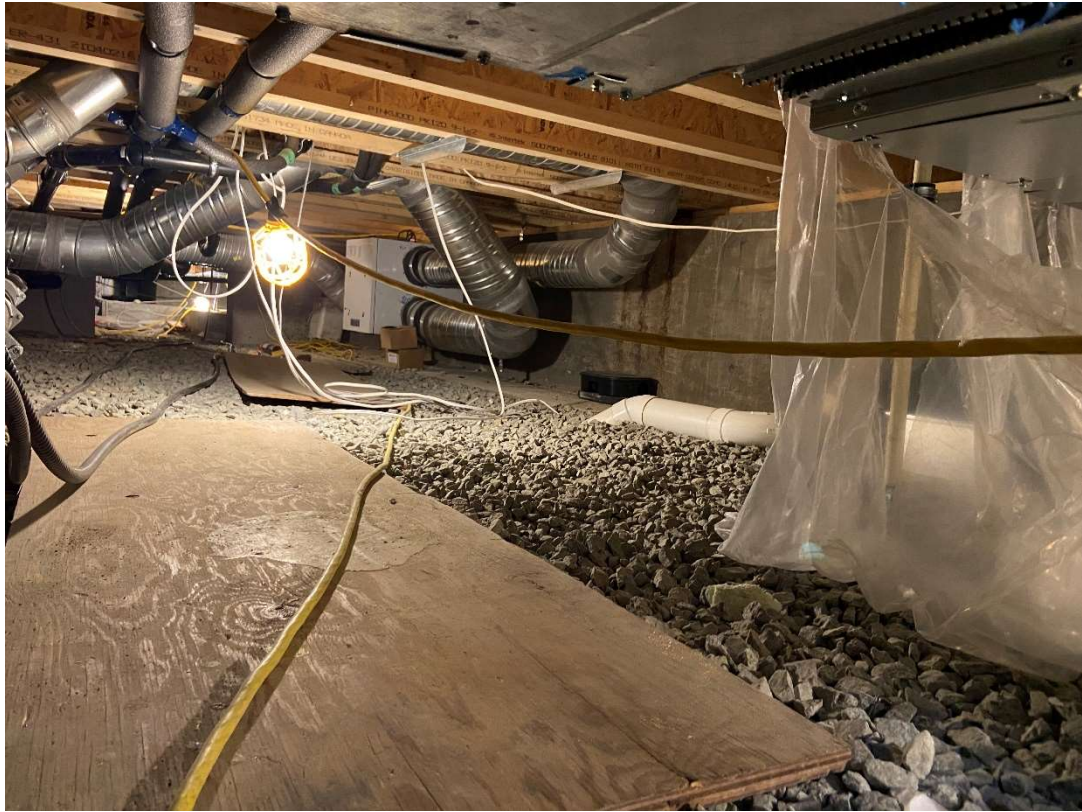
Photo 13: Crawlspace under addition
