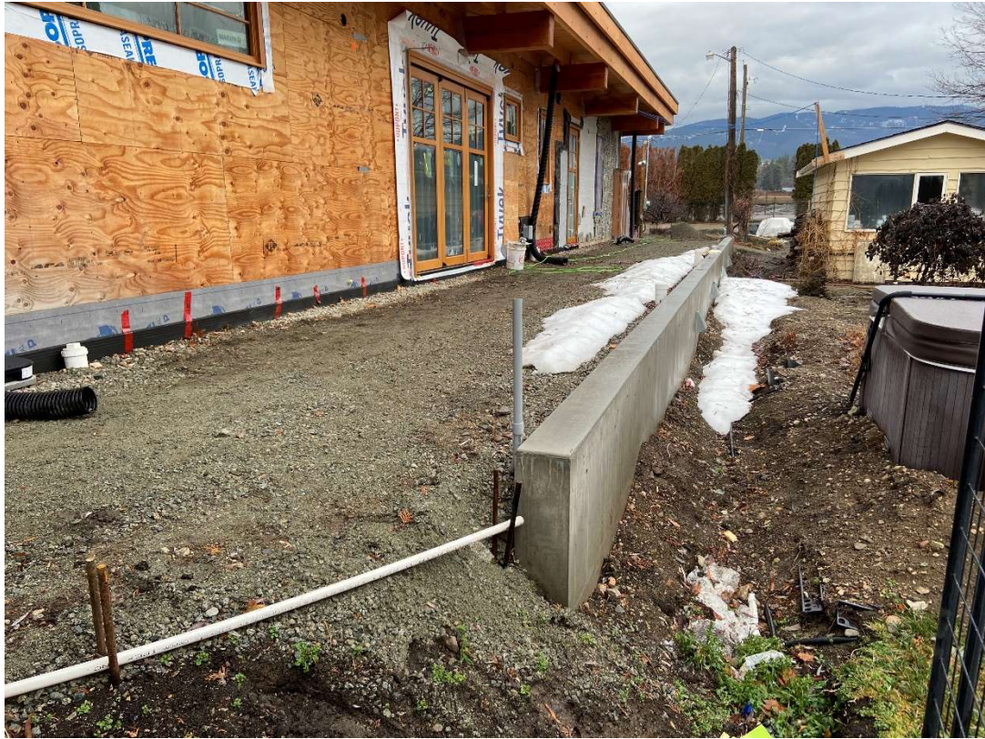
Photo 7: looking north along retaining wall
