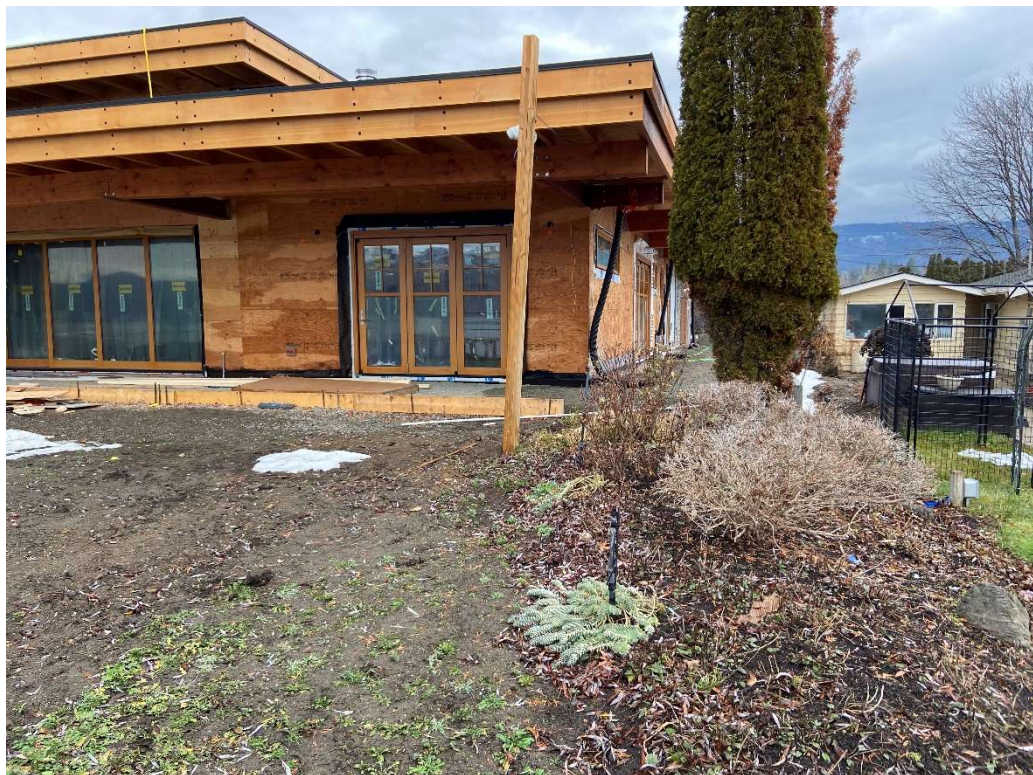
Photo 6: looking north along east side of dwelling
