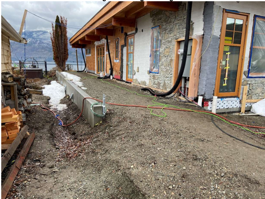
Photo 8: Looking south along retaining wall
