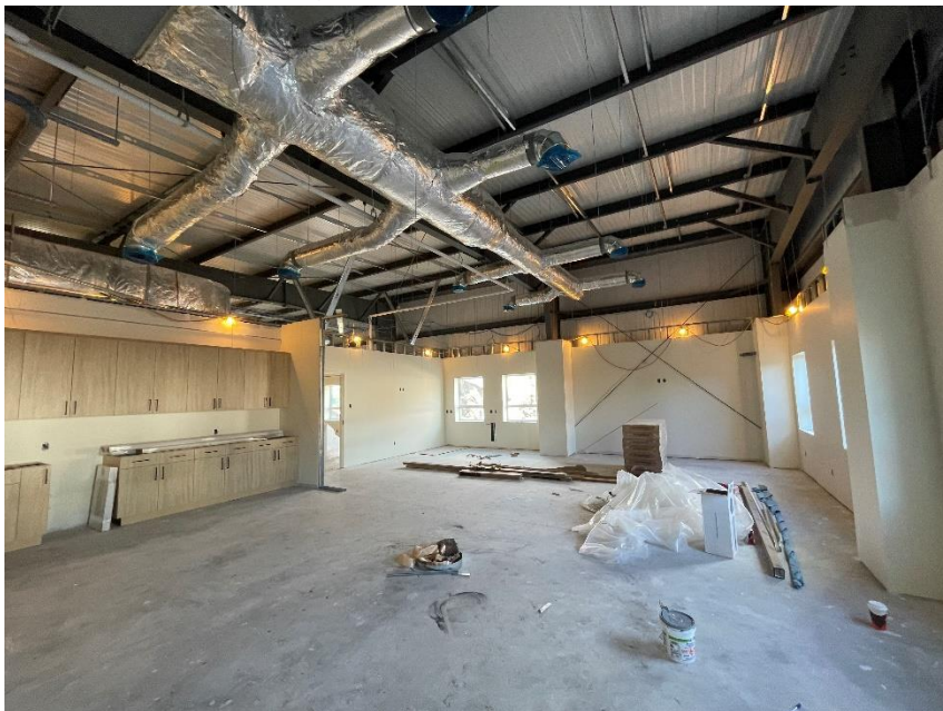
Administrative area, entrance and file room
