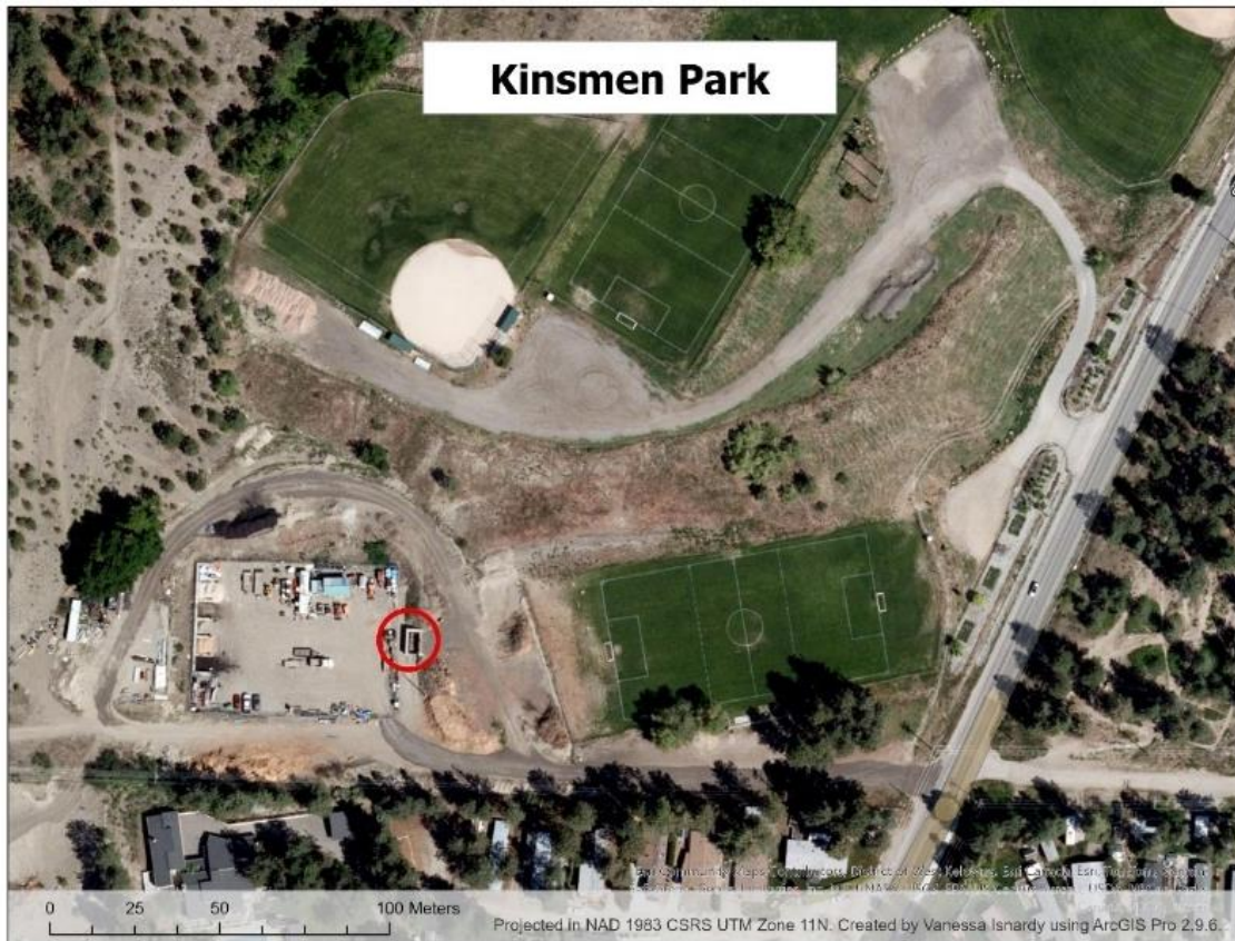
Figure 27. City of West Kelowna park staff bring garbage collected from park receptacles to an open dumpster (circled in red) located at Kinsmen Park.
