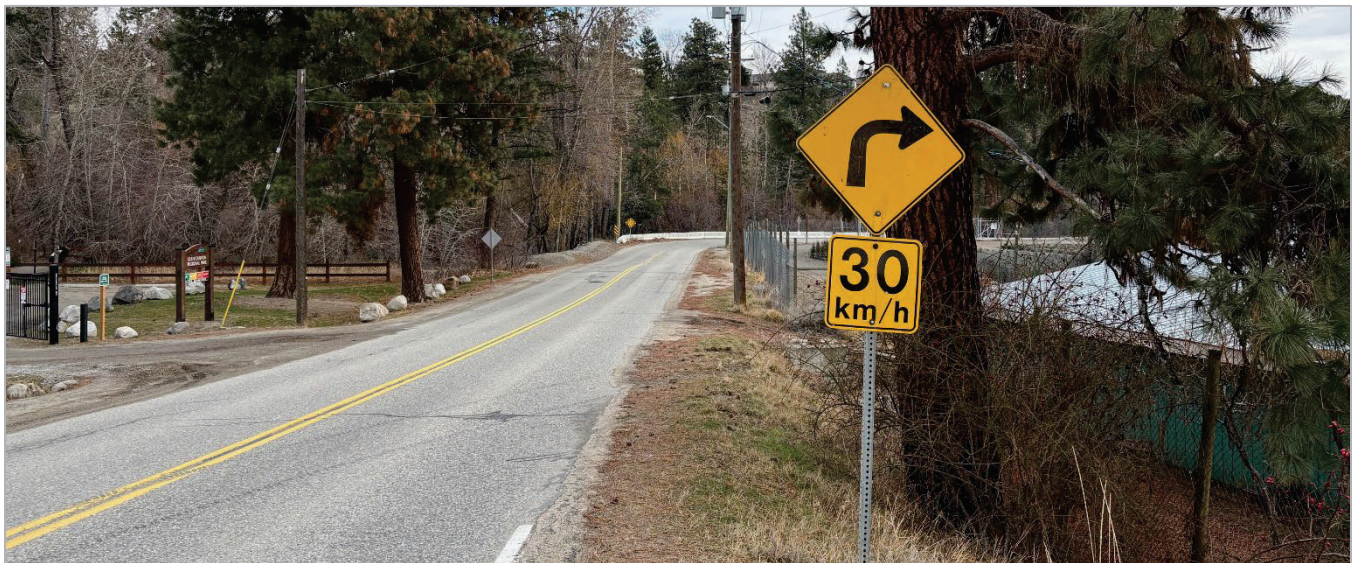
Figure 6: Curve Warning with Advisory Speed Located Far from Curve
