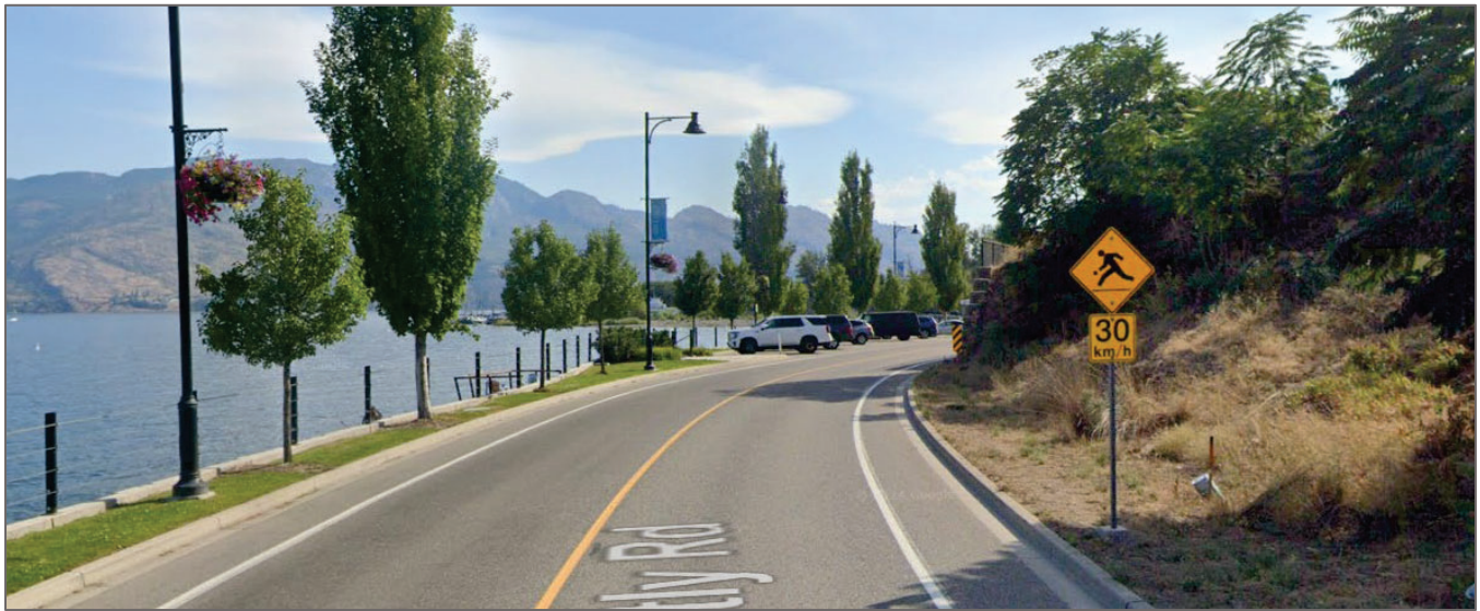
Figure 3: Southbound Sightline Constraint Entering Angle Parking Segment
