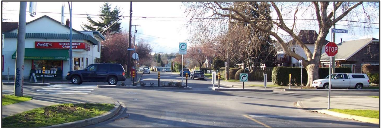
Figure 9: Raised Median through Intersection
