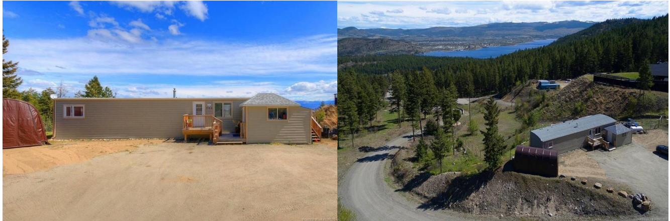
Figure 1 - Mobile Home Installed Onsite
