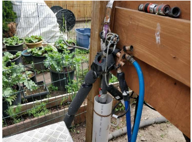
Figure 2 – Insulated Water Connection
