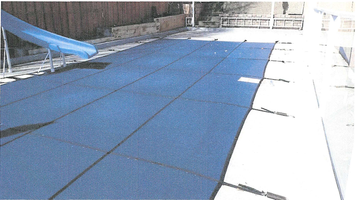
Photo 6. The owners have proposed an expansion of the pool which will extend away from the 15m setback towards the far end of the photo. The pool will be realigned with the house and formed with new concrete.
