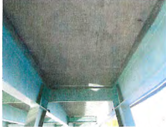
Coating (Struct): Localized loss of coating and light corrosion. Edge defects and chalking of coating throughout. Bird nests and droppings advancing deterioration of coating.
