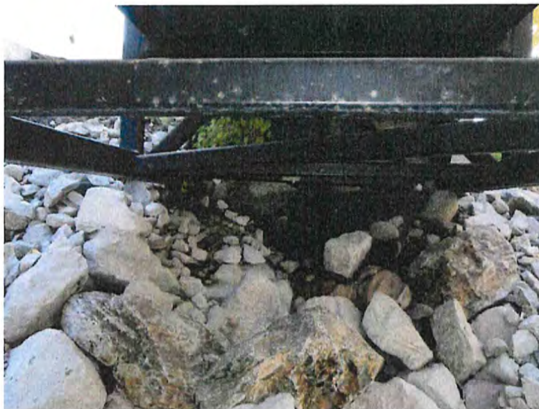
Bottom Chord and Bracing – note minor corrosion
