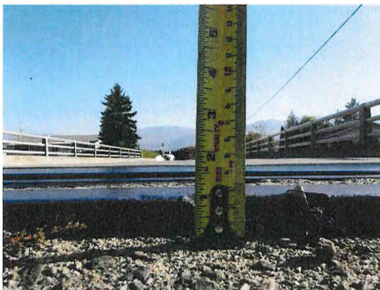
Deck joints - 38mm gap and 25mm grade differential at West deck joint. 28mm gap at East deck joint. East angle plates minor debonding across 75% for deck width.
