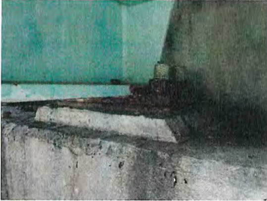
Bearings: Localized medium/severe corrosion and section loss on exterior girder bearings. Pack rust creating separation between bearing plates.
