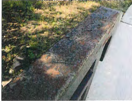
Coating (Railings): Localized light corrosion with no section loss.
