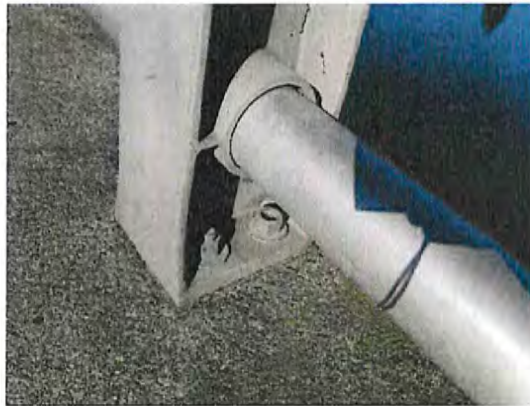
Railing Parapets: Guardrail splice bolts missing on east guardrail. Several guardrail post bolts only partially threaded.
