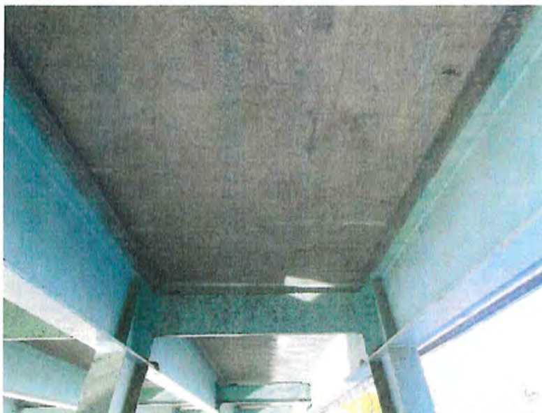
Coating – note coating defects throughout, with localized loss of coating, light corrosion and bird nests/droppings
