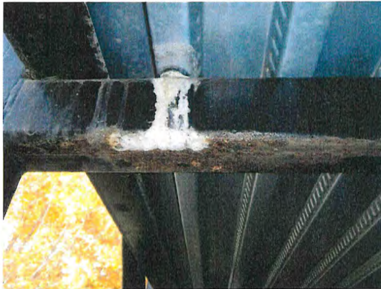
Typical Diaphragm – note staining and corrosion
