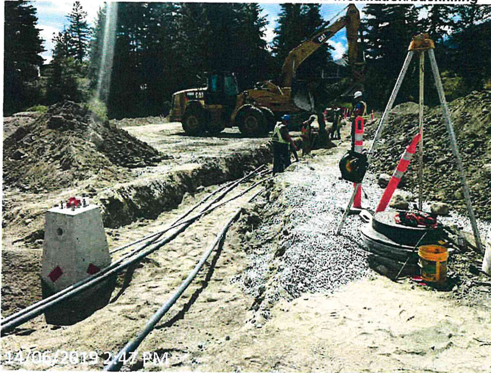
Figure 3 – Irrigation line installations in progress
