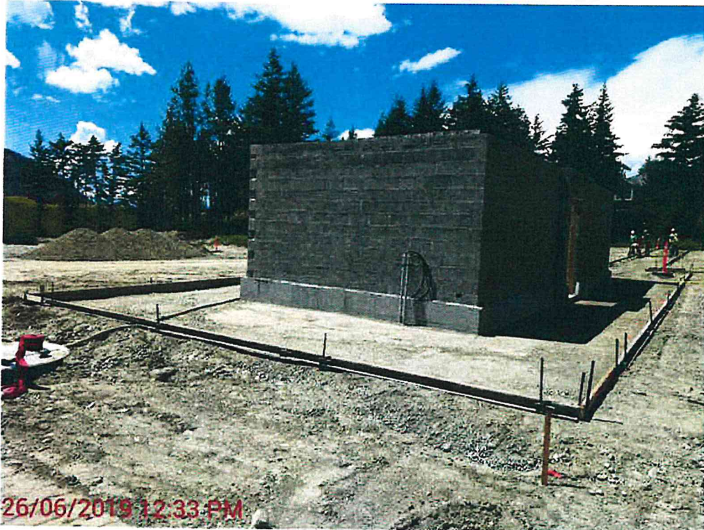
Figure 5 – Concrete forms for washroom pad and sidewalks before concrete pour, Lift Station (left) now buried
