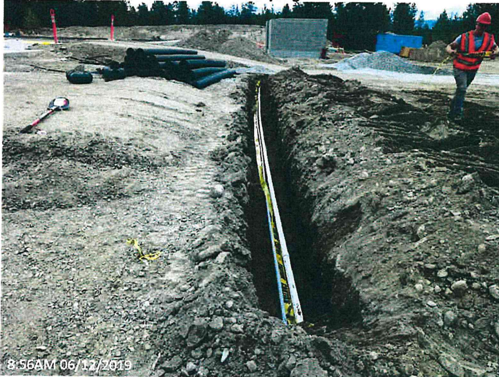
Figure 3 – Irrigation line installations in progress
