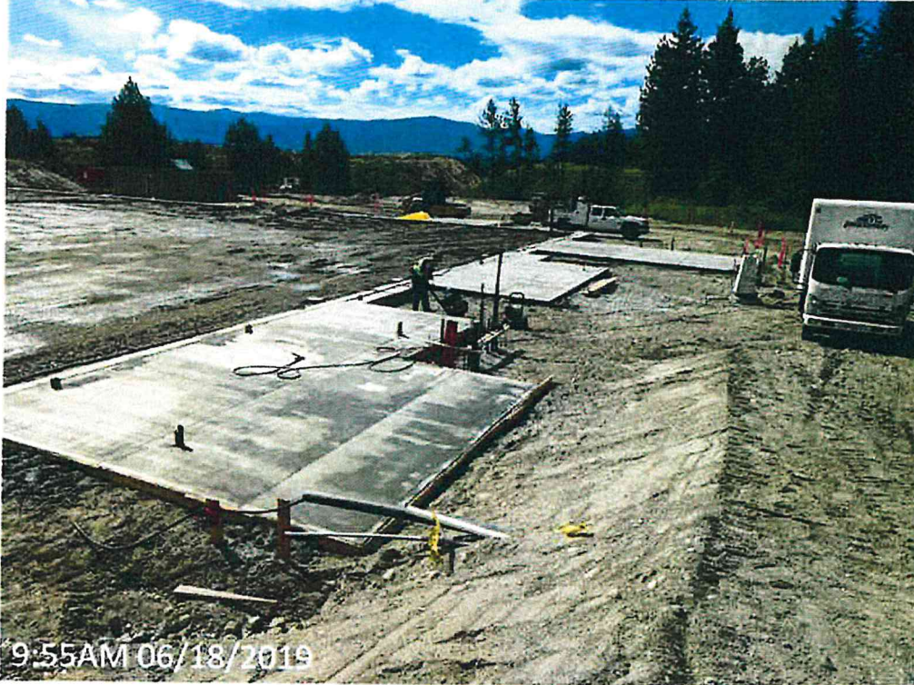
Figure 5 – Concrete forms for washroom pad and sidewalks before concrete pour, Lift Station (left) now buried
